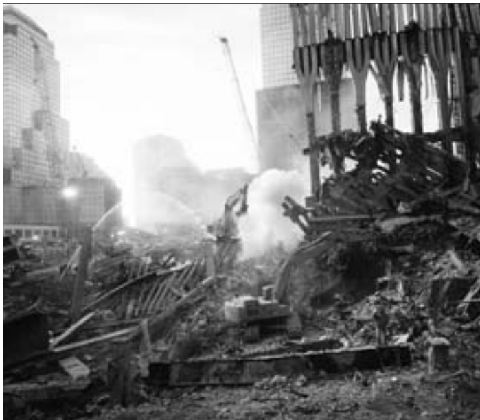
October 24, 2001. Inside the pile looking west.
